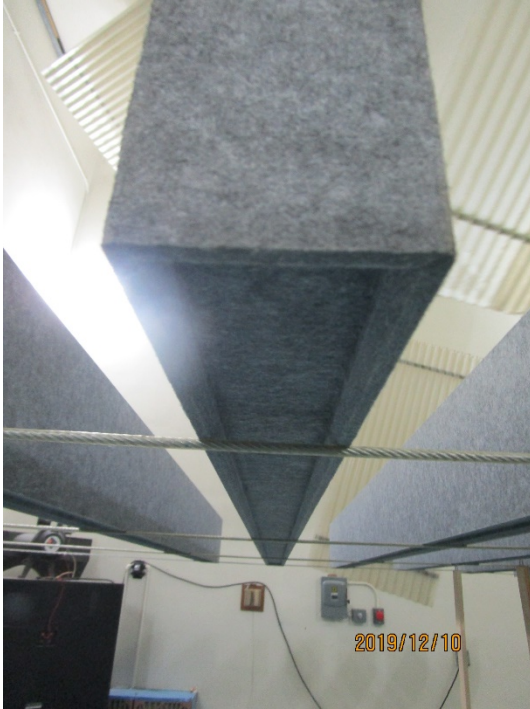
Figure 3 – Underside of individual baffle
