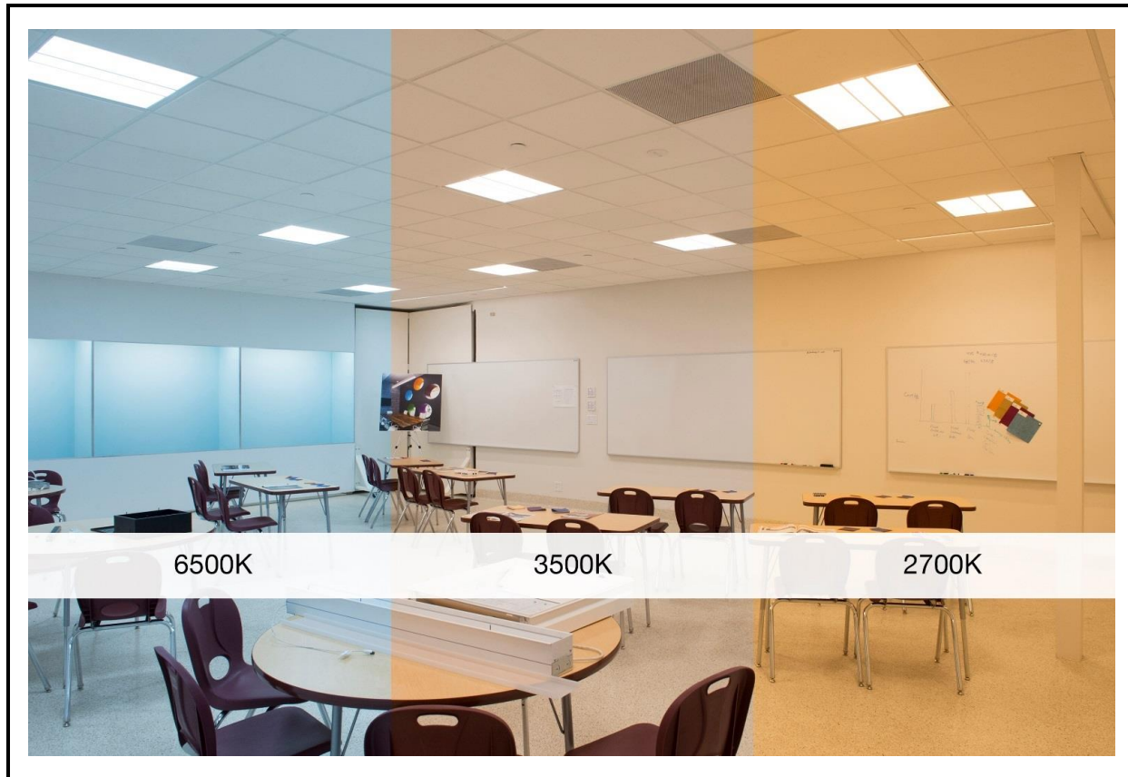
Figure 4.18 Composite Picture of the Completed NICLS Technology Demonstration Site Tuned to Three Different CCT values.
