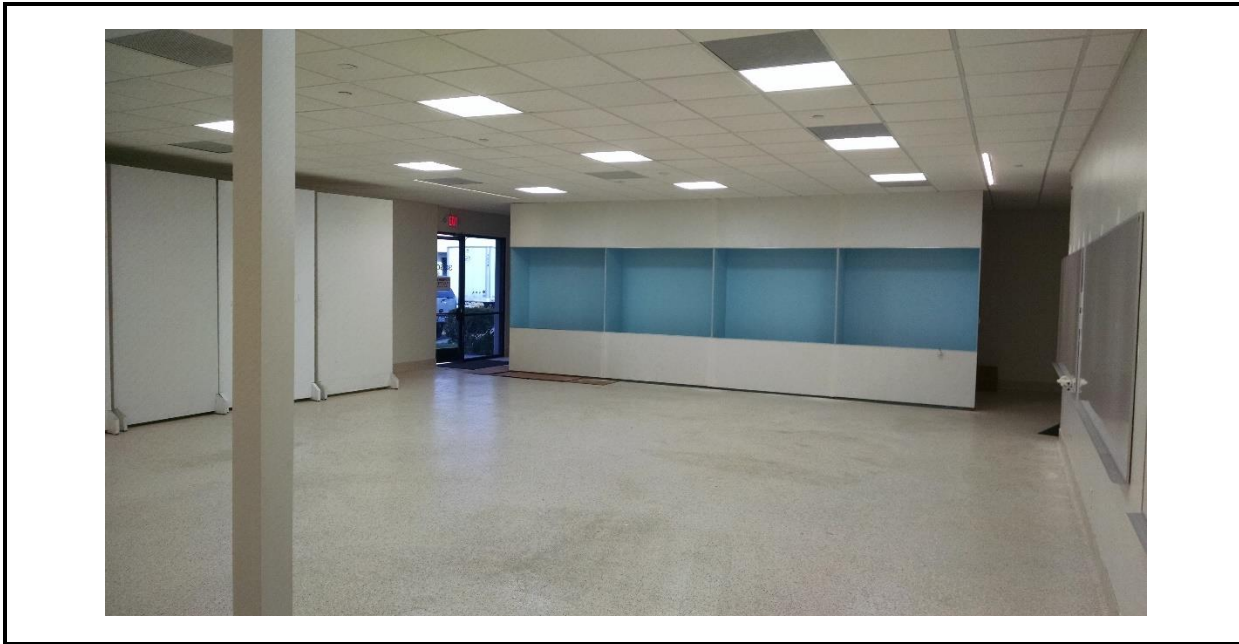
Figure 4.16 Picture of the NICLS Technology Demonstration Site for the DOE COF during Construction.
