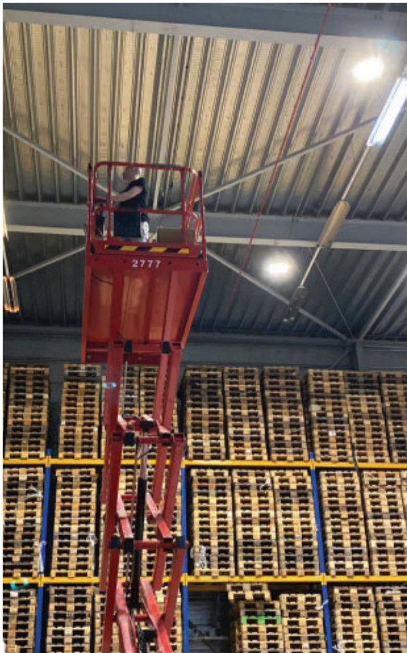
Above: Technicians install wireless controls connected via the Cosmicnode system at a warehouse in the Netherlands.
