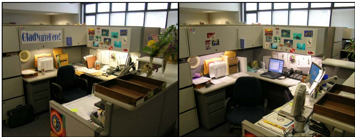
Figure 17. Example cubicle lighting at the Department of Mental Health inside the Bateson Building with former undercabinet T8 fluorescent lighting (left) and new PLS (right).
