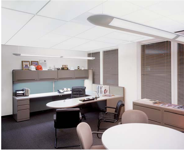
Figure 6. In this large private office primarily indirect lighting keeps vertical surfaces bright white. Task lighting mitigates shadows created by obstructions.
