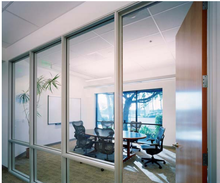
Figure 3. Here, the glass partition separating the conference room from the adjacent open office allows workers access to views and the dynamic qualities of daylight.
