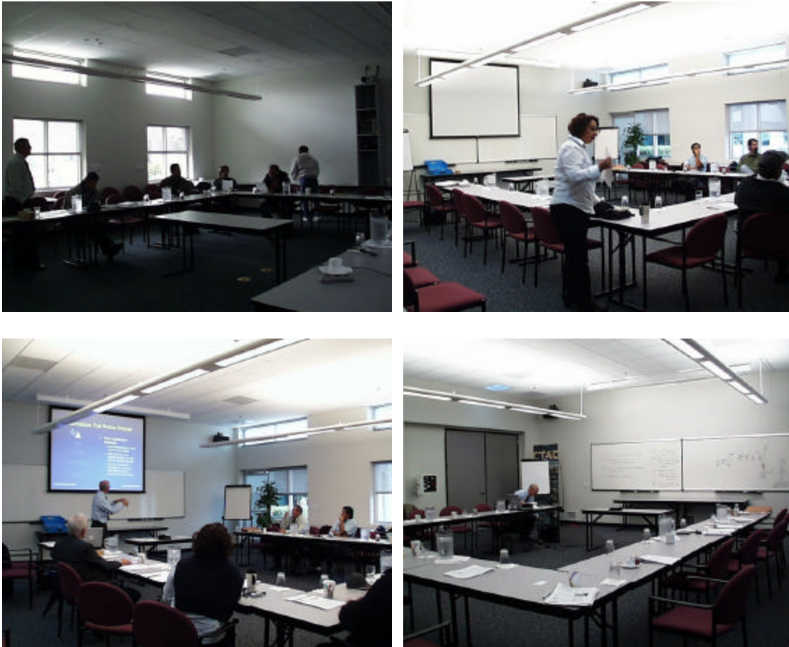
Figure 7: Pictures of lighting scenarios at the CTAC classroom. Starting at the top left is daylight only; Top right is T-5HO lighting system; Bottom left is T-8 lighting in A/V mode; Bottom right is T-8 lighting with whiteboard lighting on.
