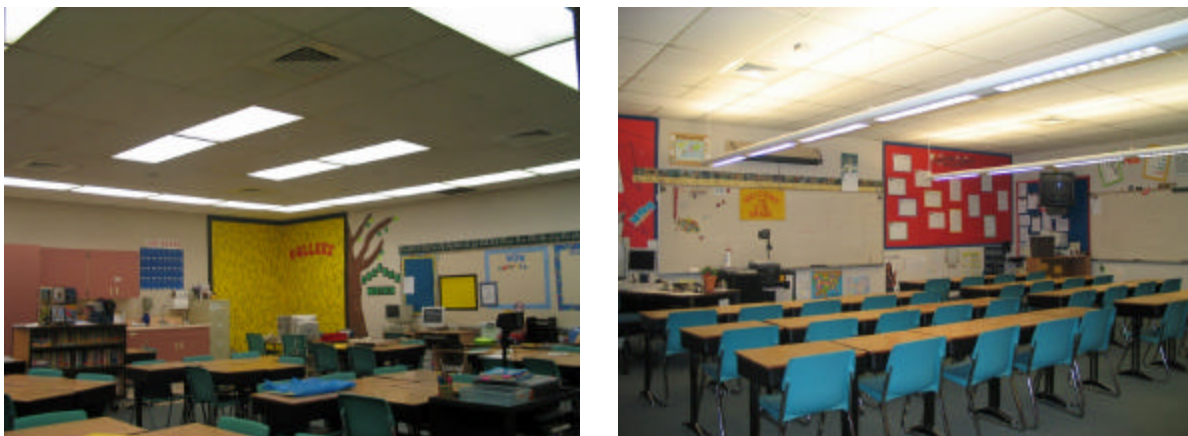
Figure 1: Existing Lighting System (1.8 Watts/ S.F.) and New ICLS System (.8 Watts/ S.F.)
