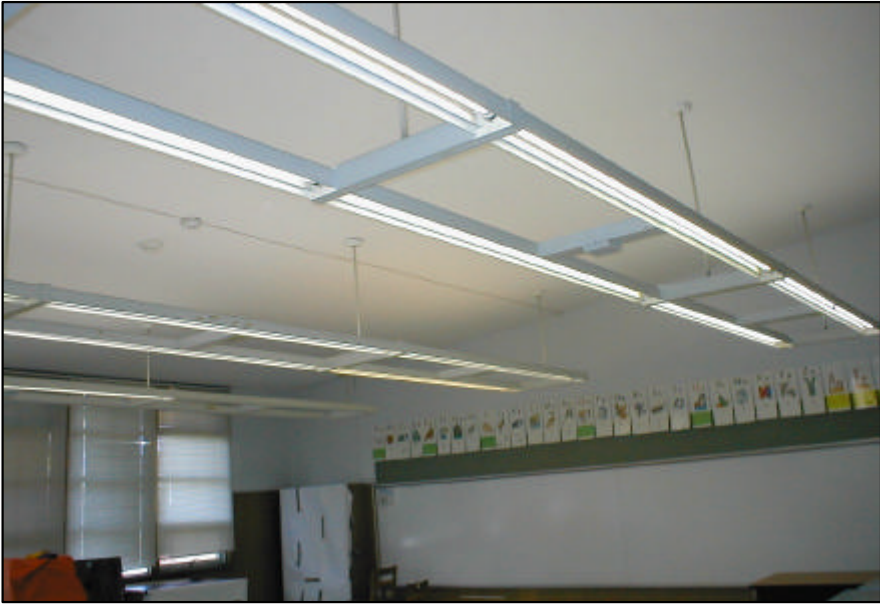
Highland Elementary Control Room
